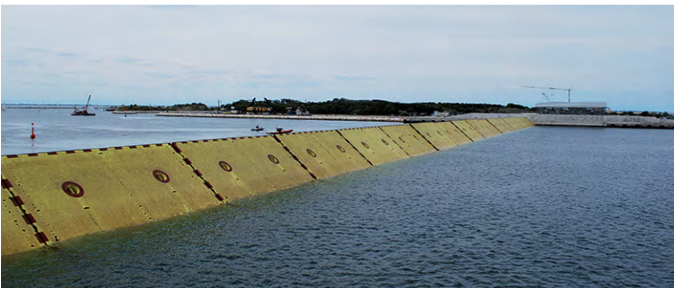
The floodgates being manoeuvred into position at the entrance to the port of Chioggia.
