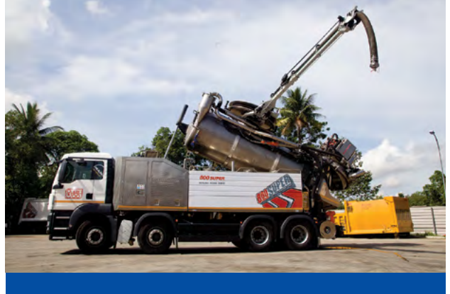
Specialised trucks are used to desilt and flush underground drain pipes.
