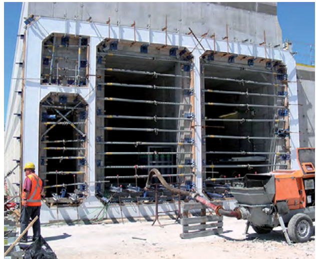
Preparing and positioning formwork on the caissons before pumping MAPEFILL MF 610.
