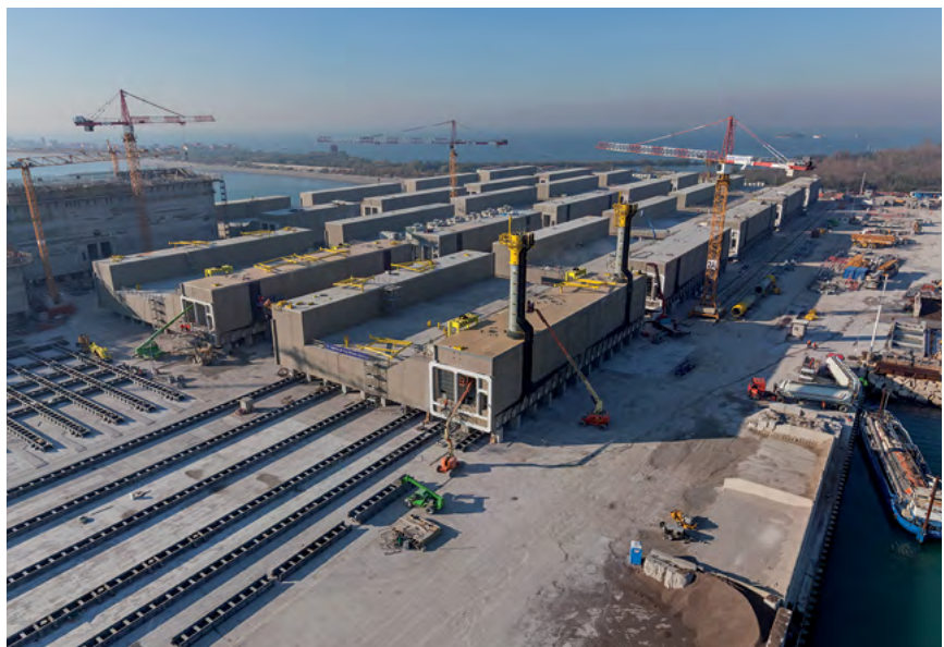
The Malamocco site where the precast concrete caissons were manufactured.
