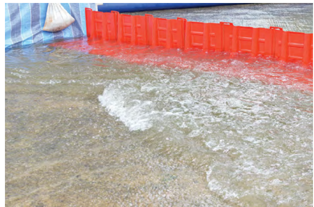
The Portable Flood Barrier (PFB) is self-anchoring and can be used on firm surfaces such as roads and pavements.
