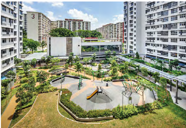
Residents can enjoy the myriad of communal spaces at St George's Towers. Image: LOOK Architects.
