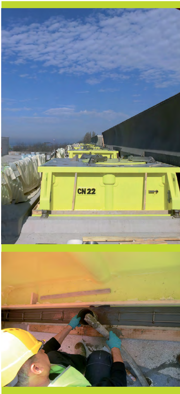
The metal floodgates are anchored to the reinforced concrete caissons with a hinge mechanism which allows them to be raised and lowered. The hinges were anchored using MAPEFILL MF, an expansive, fluid mortar especially designed for this site.
