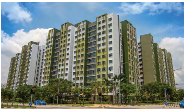
Customised large panel slabs were utilised to reduce the installations required in the Meadow Spring @ Yishun project. Image: BHCC Construction.
