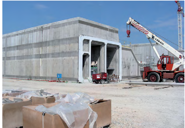
Reinforced concrete caissons being manufactured for use in the Mose project. The joint housings for the caissons were connected together with a jointing system made with MAPEFILL MF 610.
