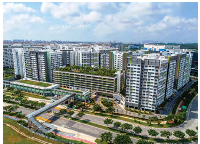
The use of collaborative technological platforms raised construction productivity in the Tampines GreenView project. Image: Ho Lee Construction.
